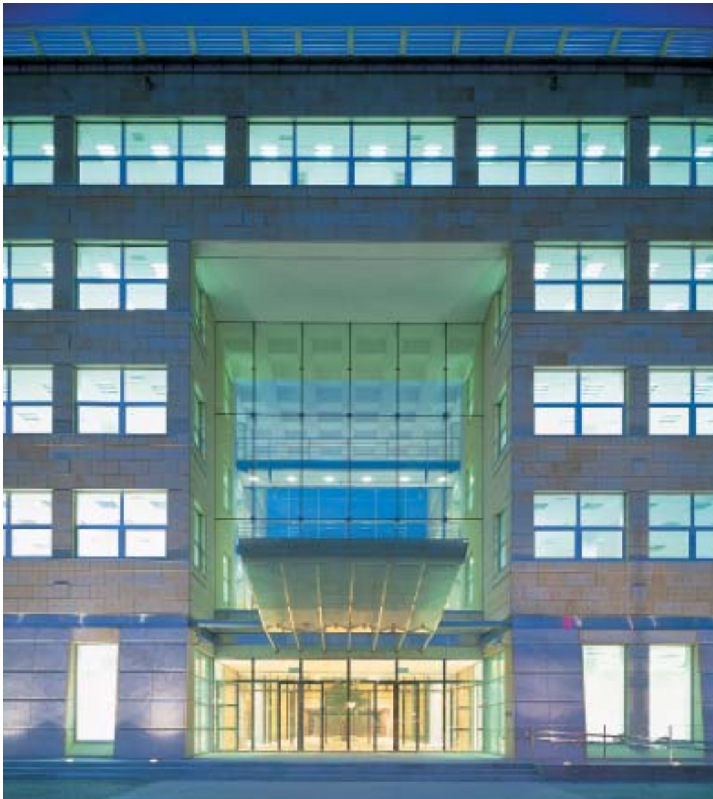
The 'mega-window', measuring 10.09 x 10.838 m, was implemented with the Planar™ system manufactured by Pilkington Architectural.
